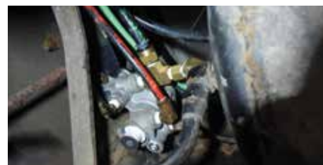
PICTURE 7 – Replacing the valve.
