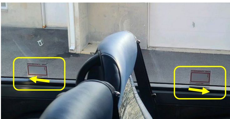
These markings, placed on a non-opening window, do not clearly differentiate between an actual emergency exit and where one can be located.
