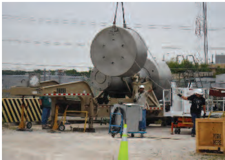
The 72B shipping cask has one of two impact limiters removed.
